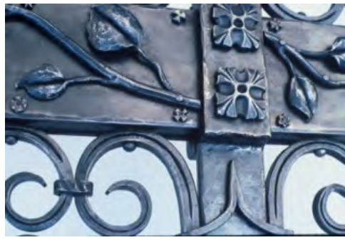
Detail of Brown Gate
